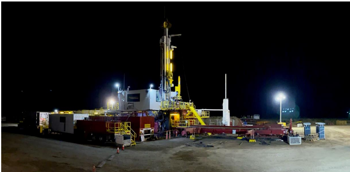
Drilling at Rougemont-2 June 2021
