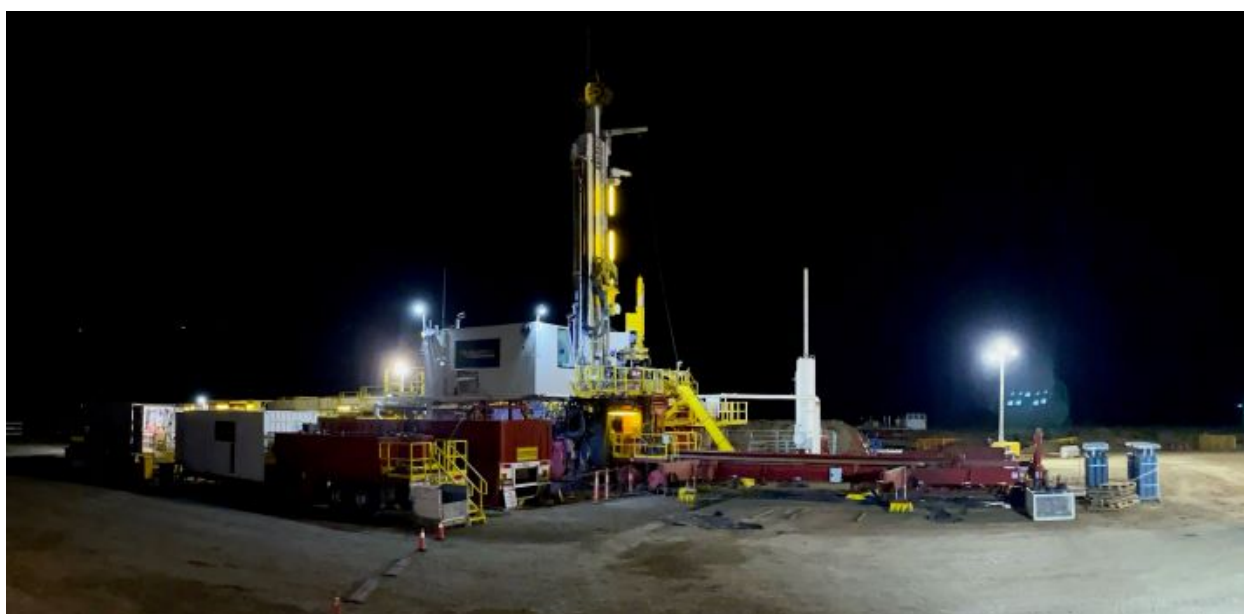
Drilling at Rougemont 2, June 2021
