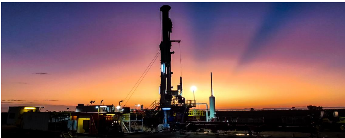
Drilling at Rougemont-3
