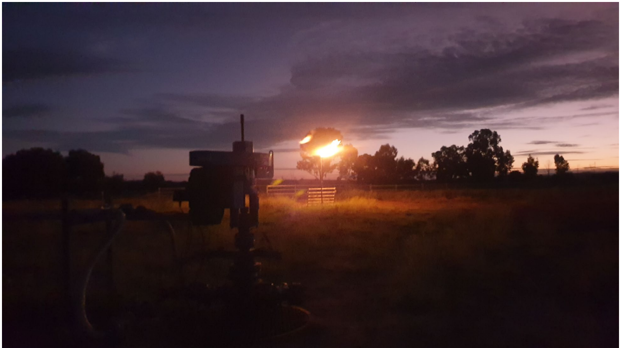
Figure: Gas flare at Rougemont-2/3 on 8 February 2023
