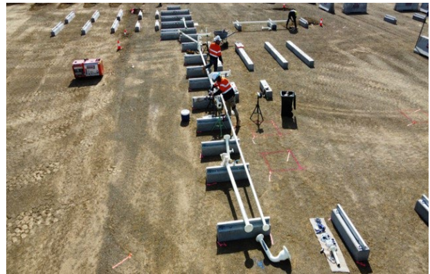
Figure 2: Mechanical crews commencing plant construction
