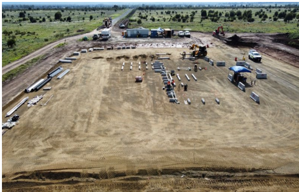
Figure 1: Completed CNG Facility pad
