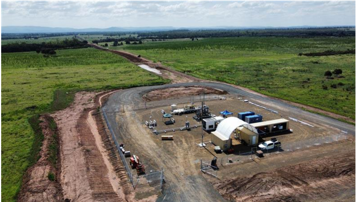
Figure 4: Full site with Rougemont 2/3 gathering system connection to the top of image. Surface rehabilitation of corridor and area surrounding facility pad well underway and benefiting from recent rain.
