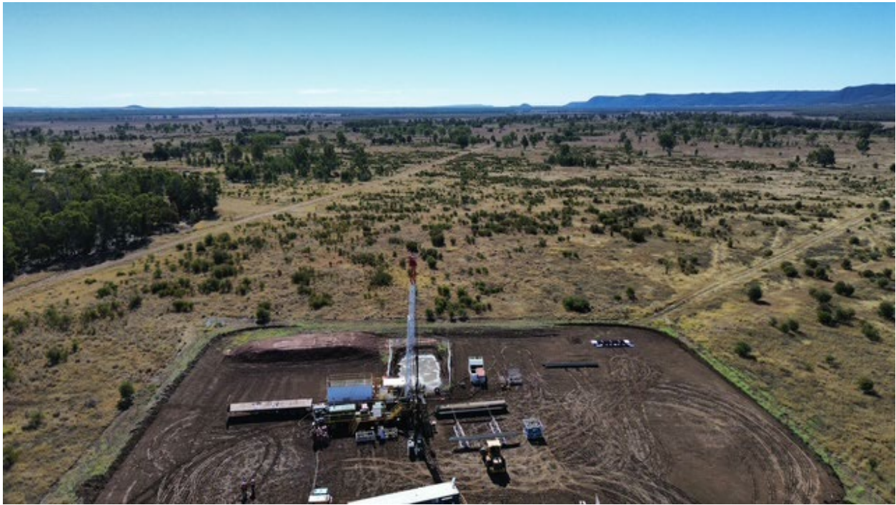
Figure 2: Workover Rig undertaking completion activities at Rougemont-6
