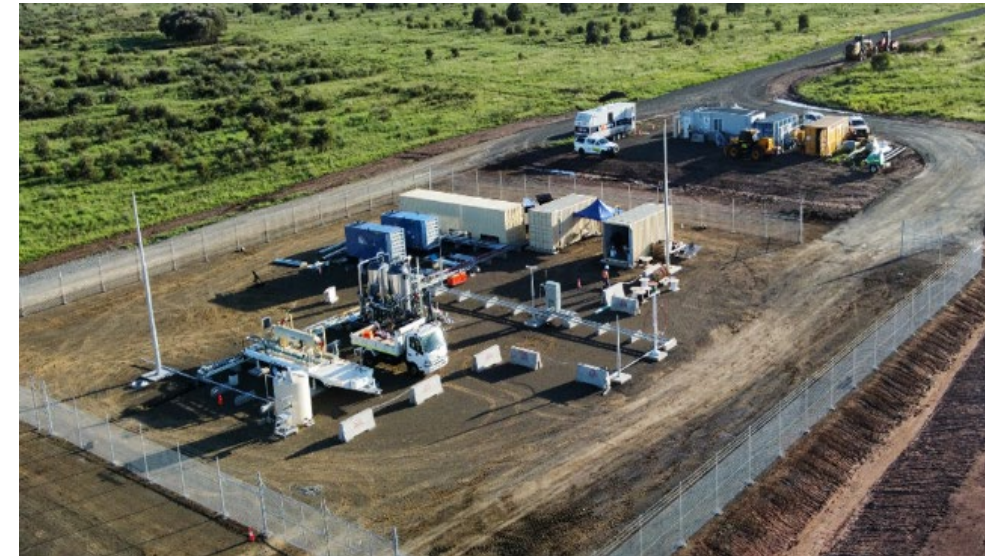
(Image) Aerial photo of commissioned HDNG plant
